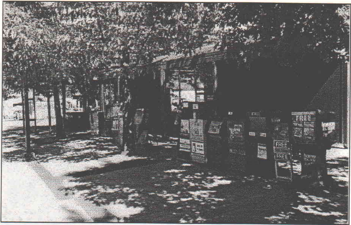
Figure 9.1. Kenmore Park-and-Ride. Shelter area.
