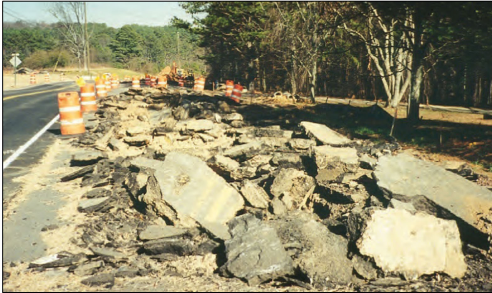
FIGURE 2. Road slabs produced from full-depth demolition (West, 2015).
