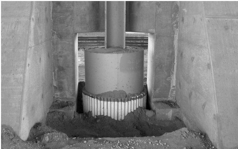
Seismic retrofitting to the Spokane Street Bridge, Seattle
