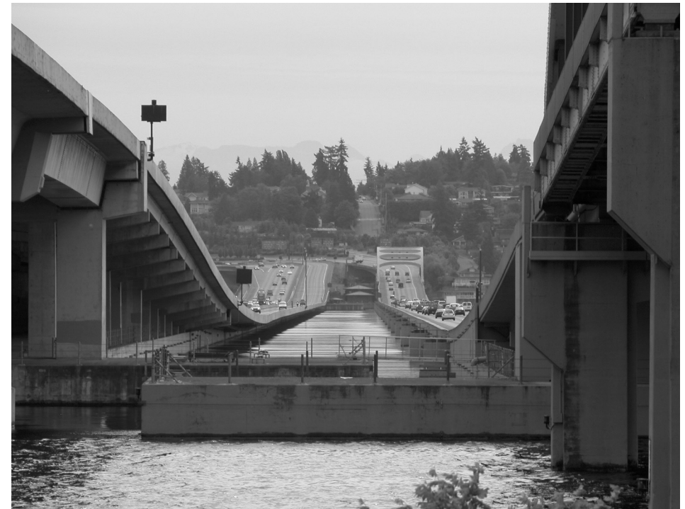
The Lacey V. Murrow Memorial Bridge, better known as the I-90 floating bridge, is one of two floating bridges that cross Lake Washington near Seattle.
