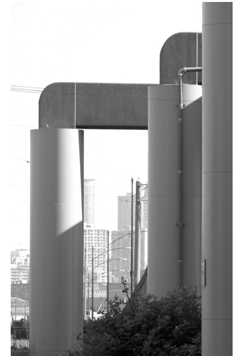
Outrigger bent and knee joint support the Alaskan Way Viaduct, Seattle.
