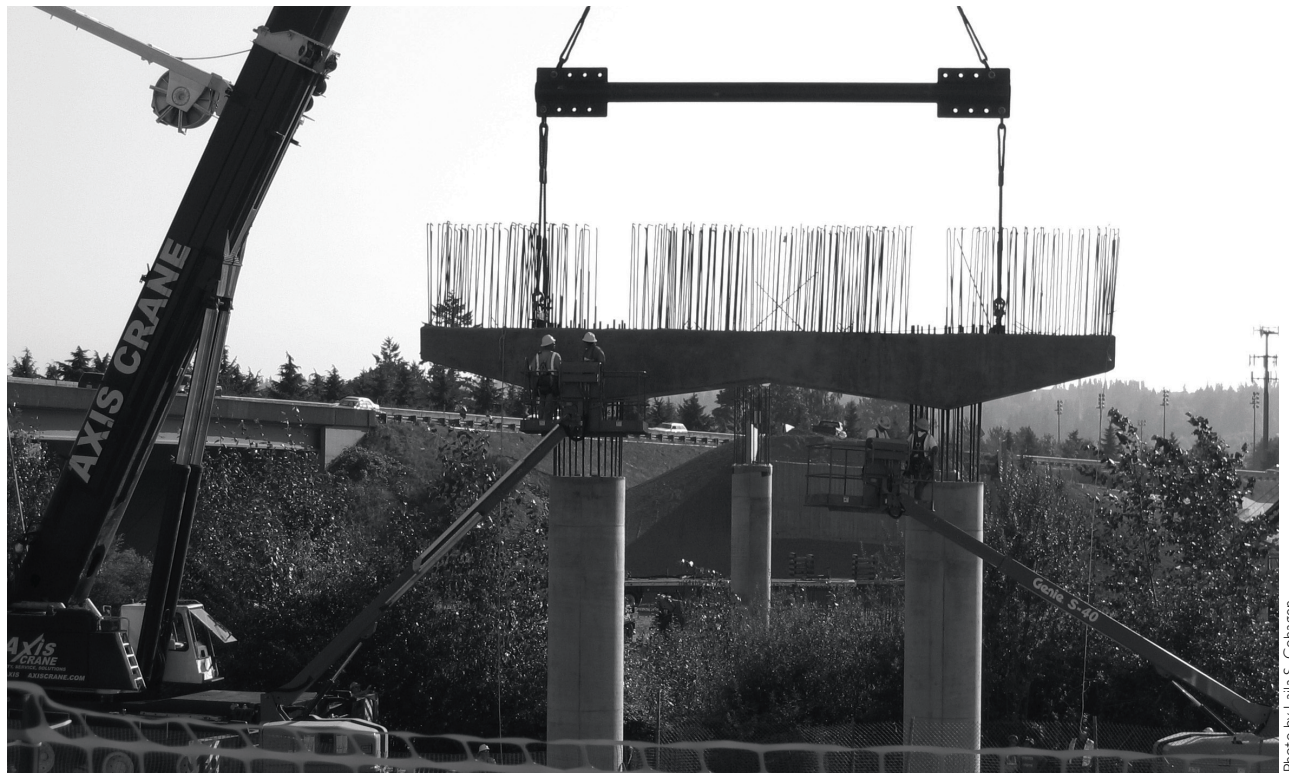
This construction on an SR 520 ramp in Redmond, Washington, is using segmental construction.
