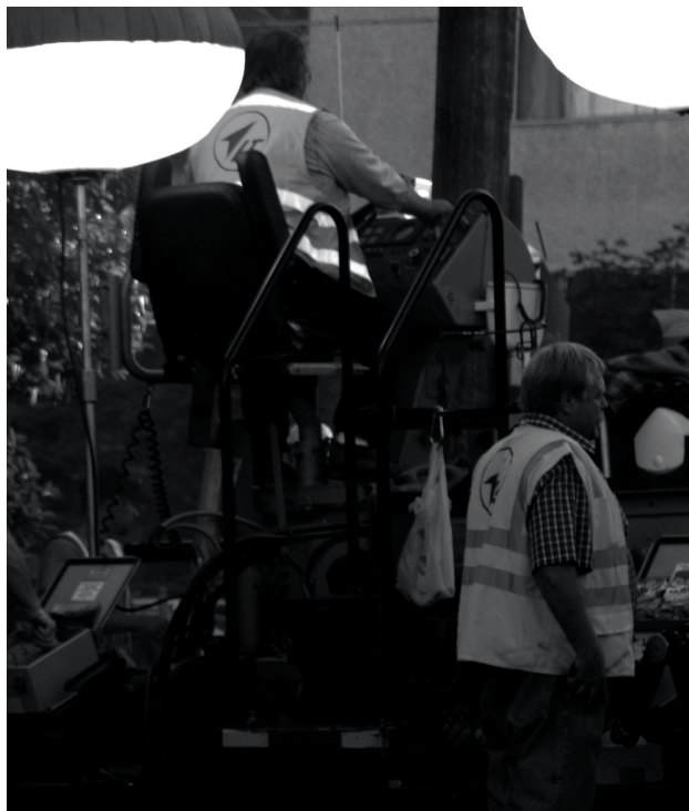
Maintenance at night may make operations more cost and time effective.
