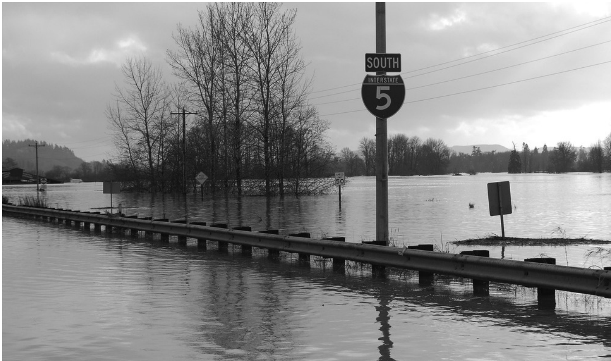
To aid WSDOT in decreasing future flood impacts in the Centralia, Washington, region, researchers evaluated the benefits that various projects to reduce flood damage would provide.
