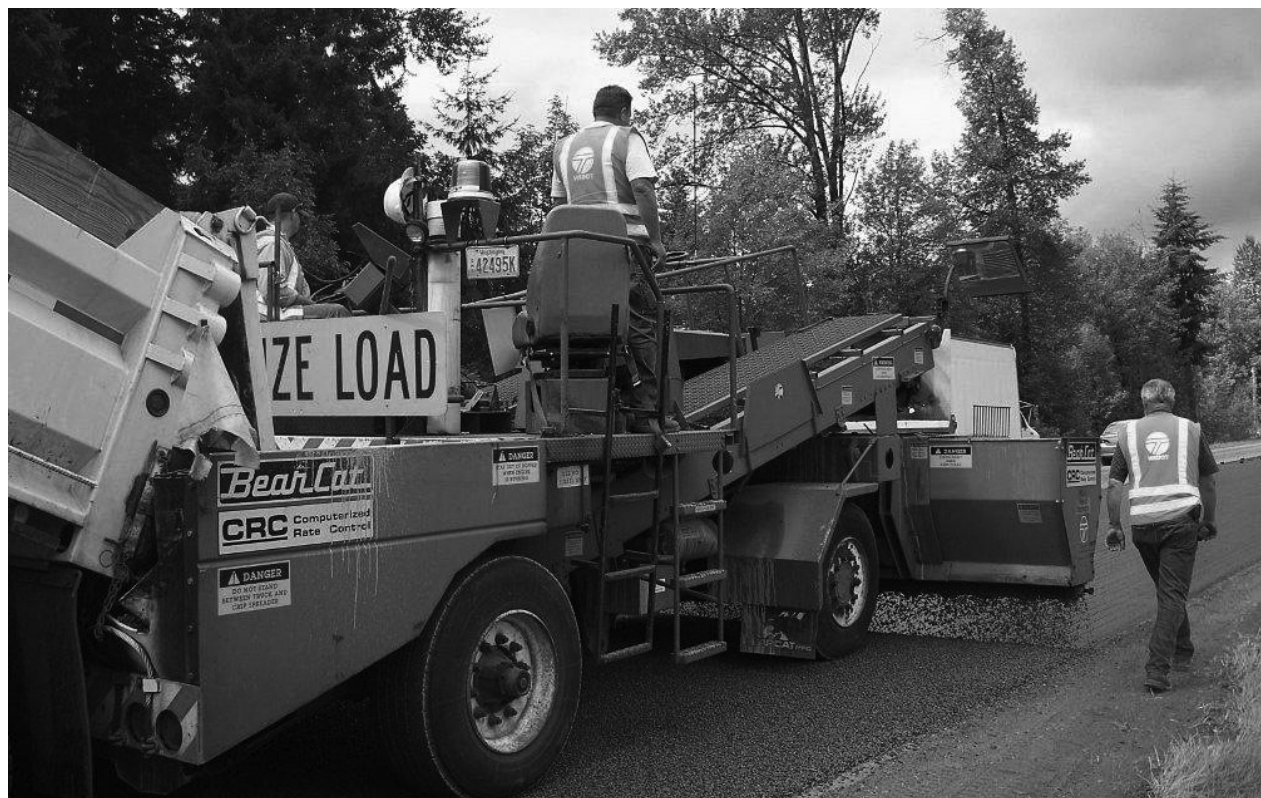
Chip seals combine asphalt and aggregate for lower cost. Researchers investigated numerous aspects of successful chip seal use.
