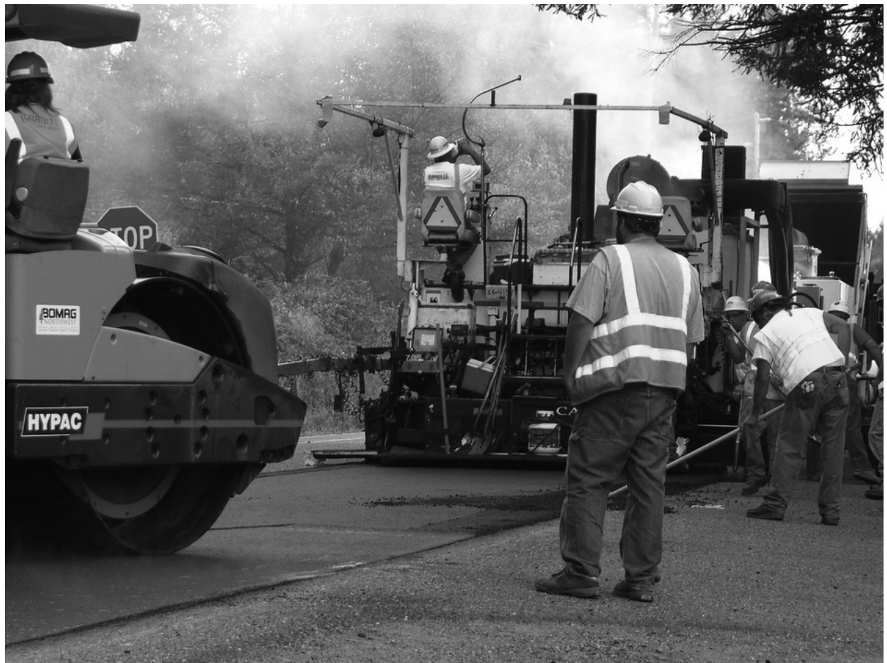
A project on optimizing hot mix asphalt performance is seeking to improve HMA surface life, particularly in Eastern Washington and the state's mountain passes.
