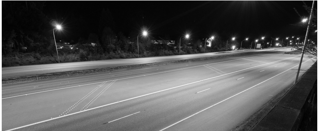
A thorough review will allow WSDOT to update its illumination design standards for installation, operation, and maintenance in order to reduce costs and improve safety.
