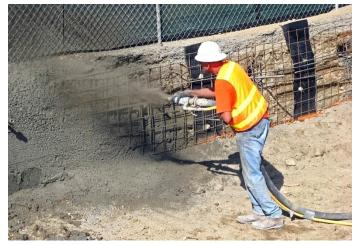
issues between the substrate and overlays. The study will develop recommendations for best practice and will test methods to assure the effective bonding and monolithic behavior of shotcrete structures for wall fascia, slope stabilization, and other applications. Read more...
