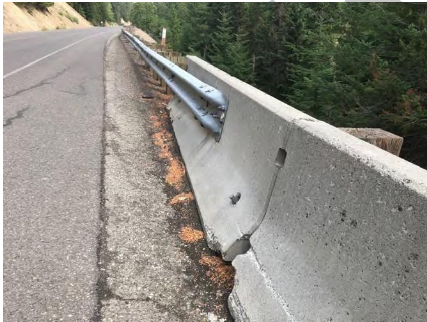
Figure 2-2. Roadway Concrete Barrier at US 12 Washington
