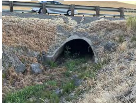
Figure 2-1. A Culvert at US 195 Washington State
