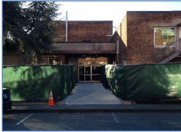
PB Building from S1 Parking
