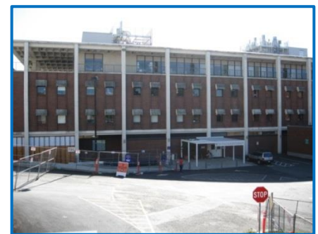
CHDD from S1 Parking Lot
