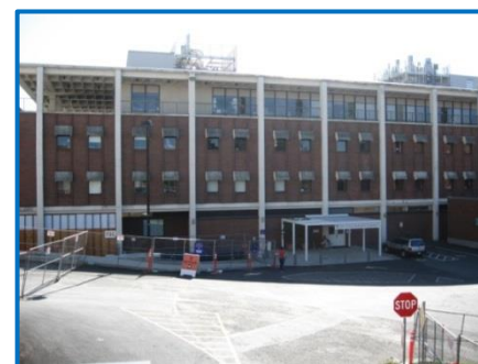
CHDD from S1 Parking Lot
