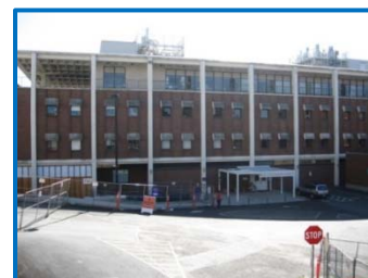
IHDD from S1 Parking Lot
