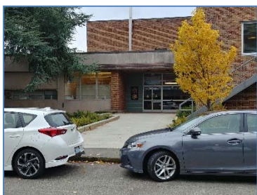
PB Building from S1 Parking
