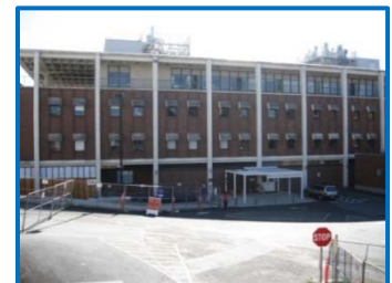
IHDD from S1 Parking Lot
