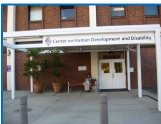
Ground Floor Entrance
