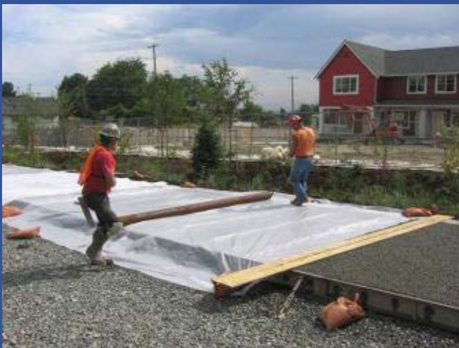
Roller for compaction
