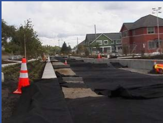
Fabric at Subgrade
