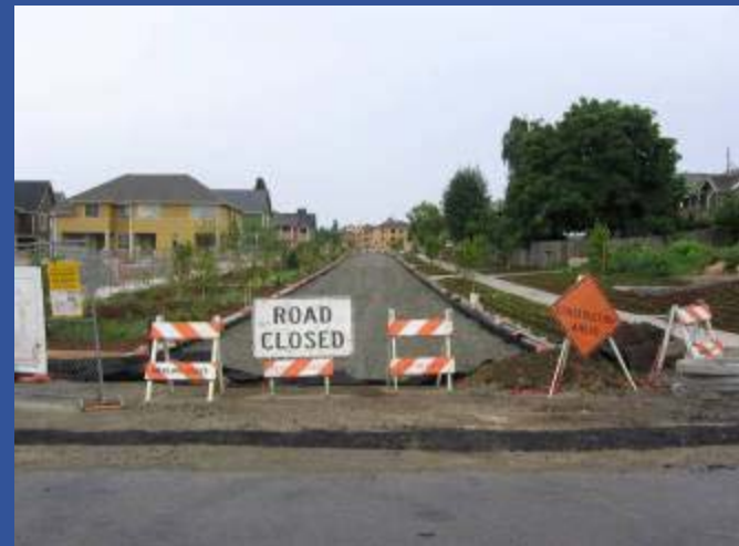
Gravel Storage Subbase
