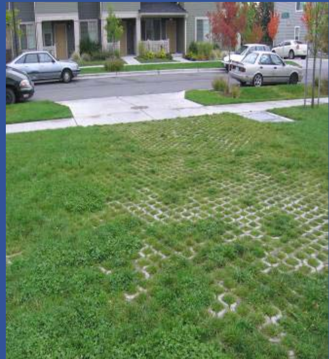
Maintenance Road using TurfStone® over 1 ½" to 2" sand and 6" of crushed rock w/o fines
