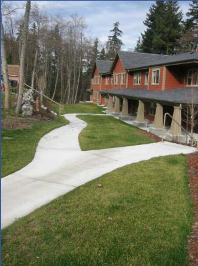
Fire lane/Maintenance road for housing site. Geoweb® Cellular Confinement system
