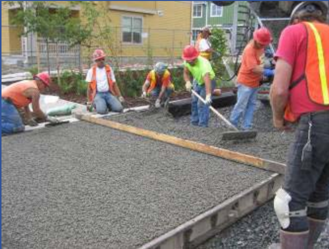
Moisten Subbase, Place Mix & Strikeoff
