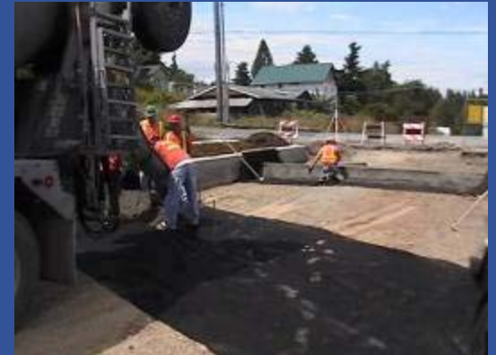
Installing Dams for Cells
