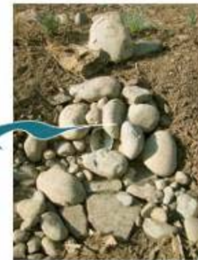
Rock lined inlet. Rock should be free of sediment, so order "washed."
