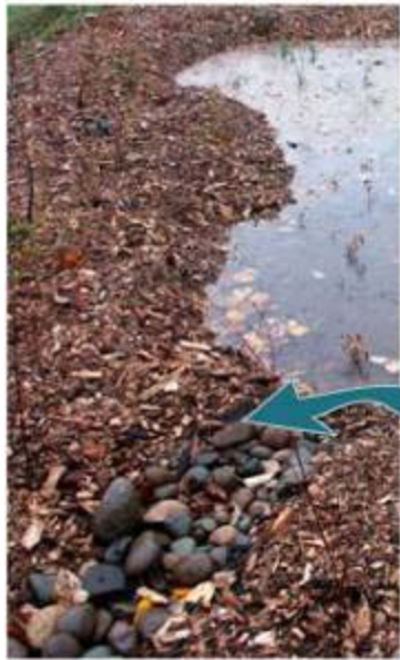
Rock lined overflow
