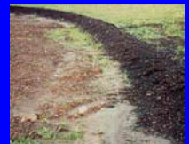
Berms instead of silt fence
