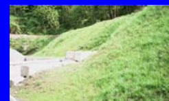
Compost blankets on steep slopes
