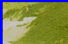
Compost blankets on steep slopes
