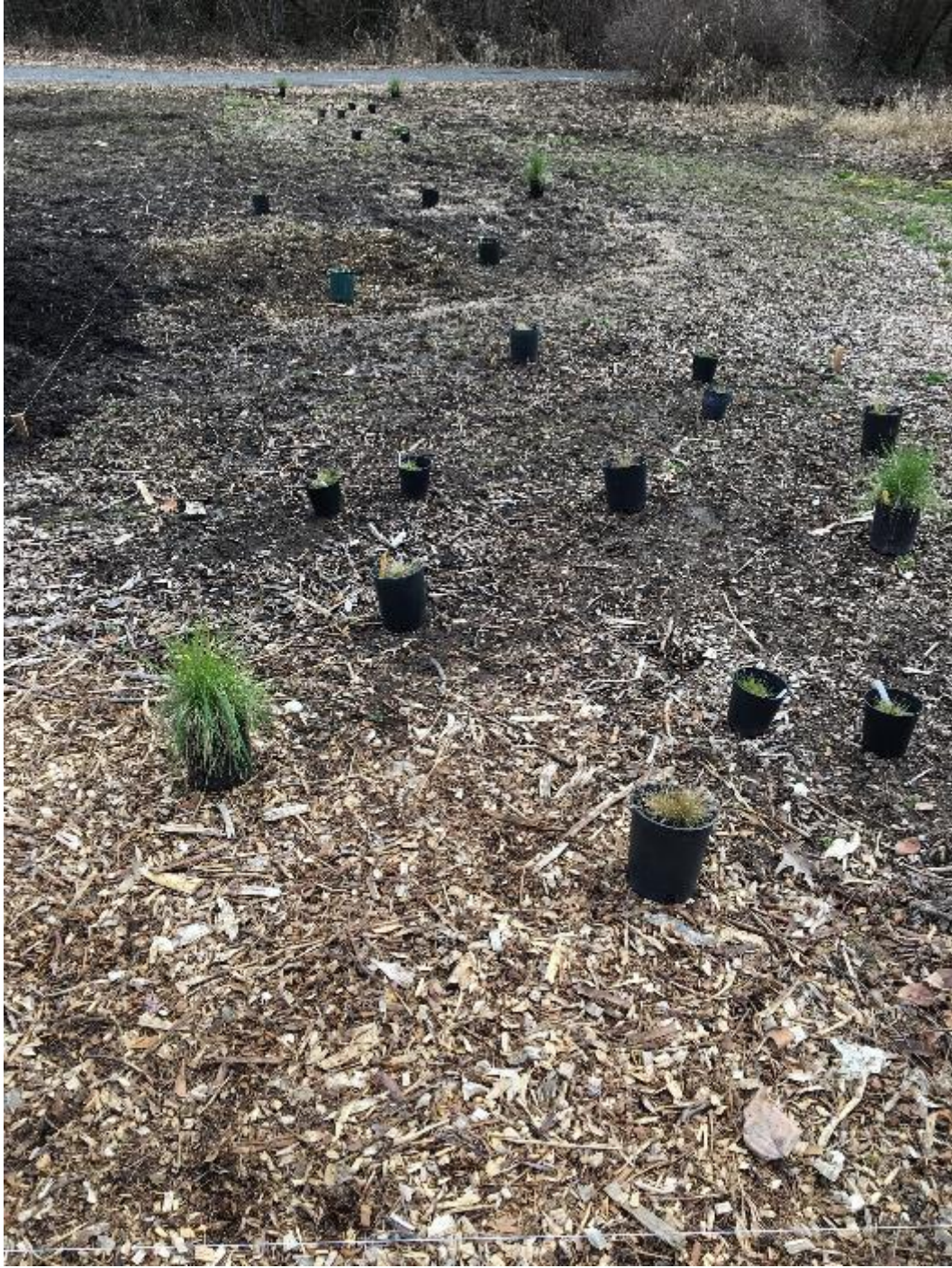
Figure 6. Staging of the plants prior to installation (Photo: A. Chan).
