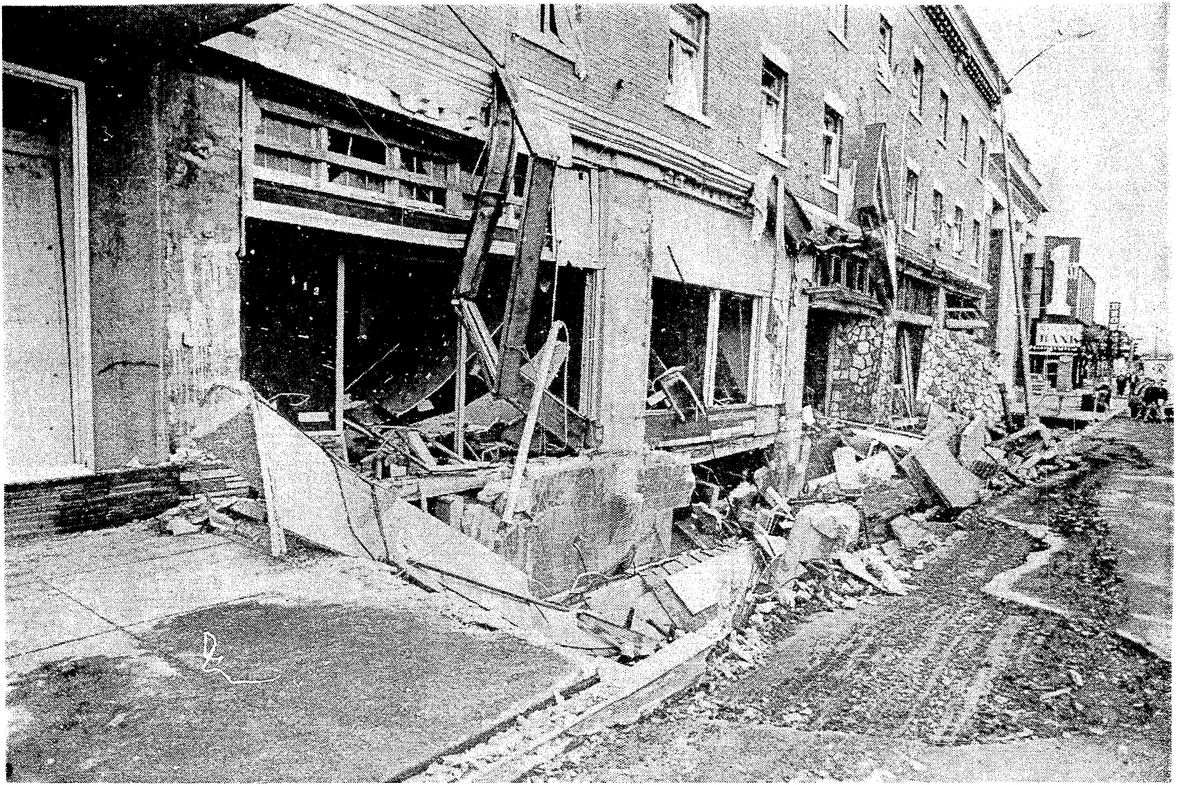
The front of a Port Angeles building was shattered and the sidewalk ripped up by last night's blast (A full page of pictures, A 3; other details and more photos, C 1.) —Staff photo by Greg Gilbert.
